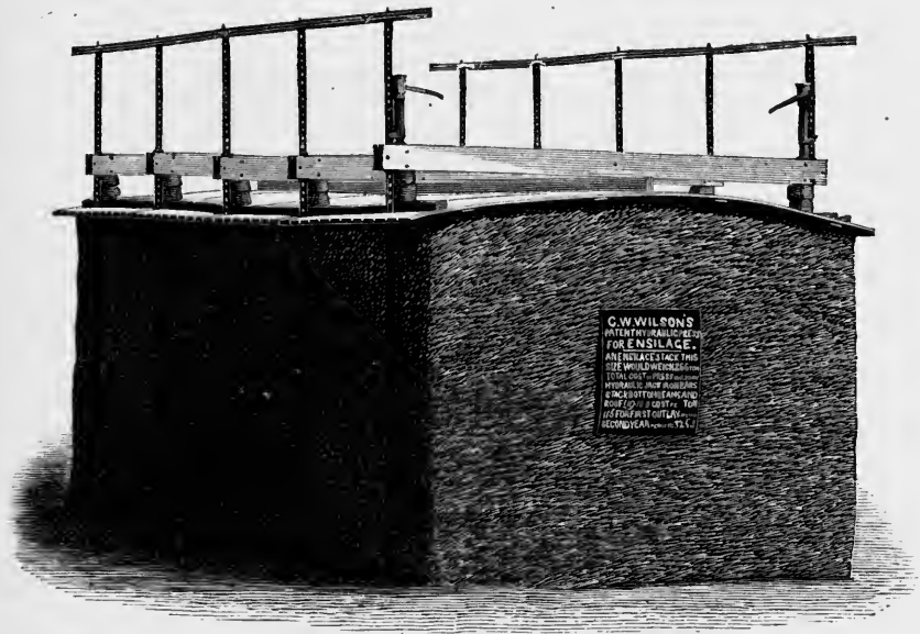
Fig. 320.—Wilson's Furcated Hydraulic Jacks as applied to Silage Stacks.
